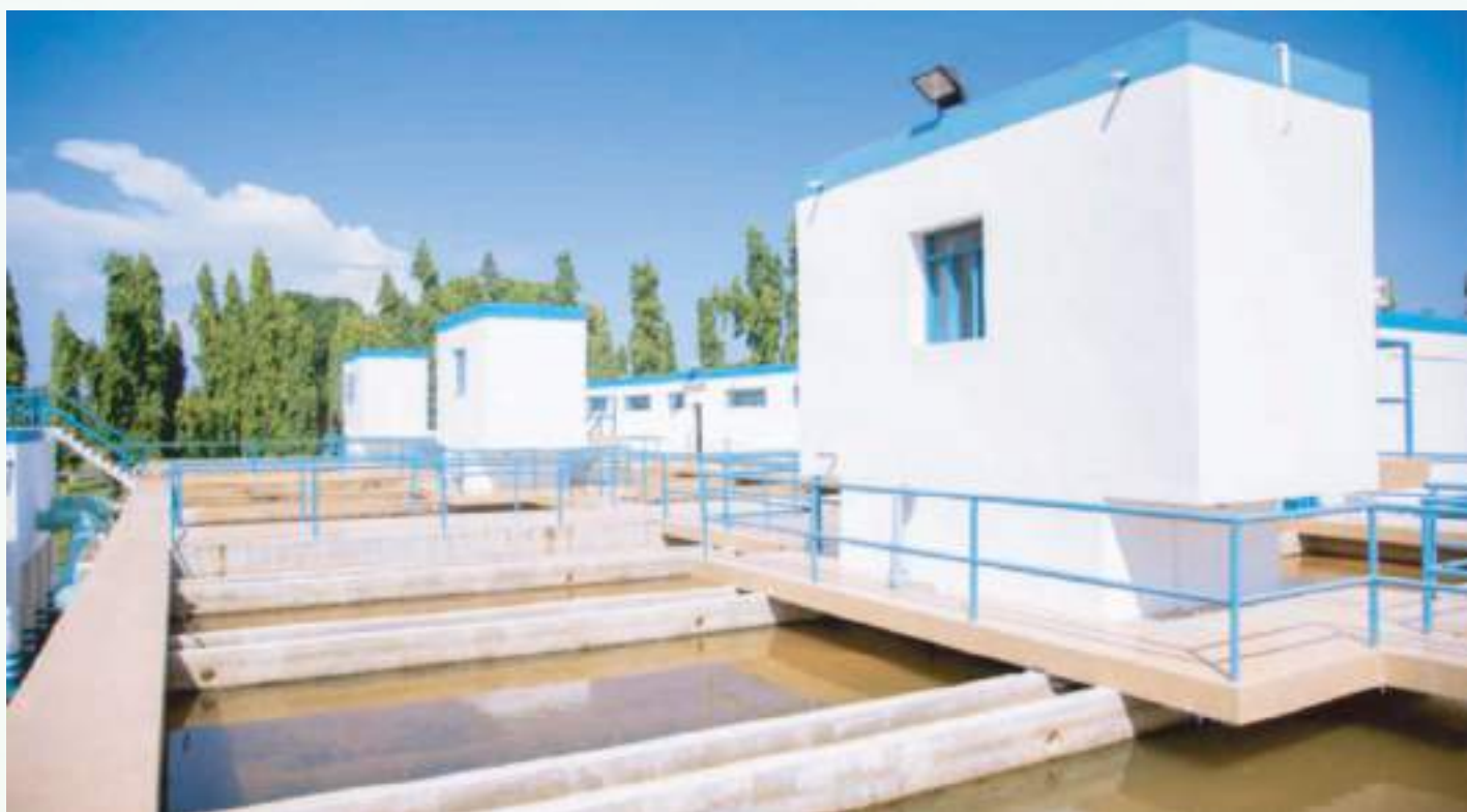
Image 1: Flocculation Tanks at Mowe Water Treatment Plant
